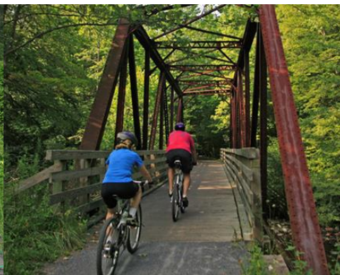
Virginia Creeper Trail, Washington County Source: Toole Design Group
